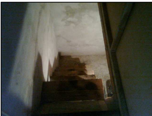
Trap in de kelder
