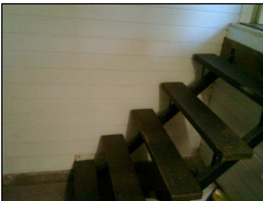
Trap in de kelder
